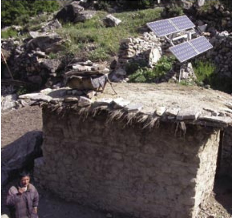
LEFT: A central PV system (300W) for 63 homes and 189 LEDs, Nepal. Photo courtesy of Alex Zahnd.
