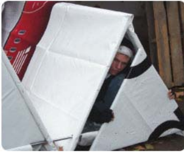
putting the doors on. doors pressure fit into the frame of structure.
