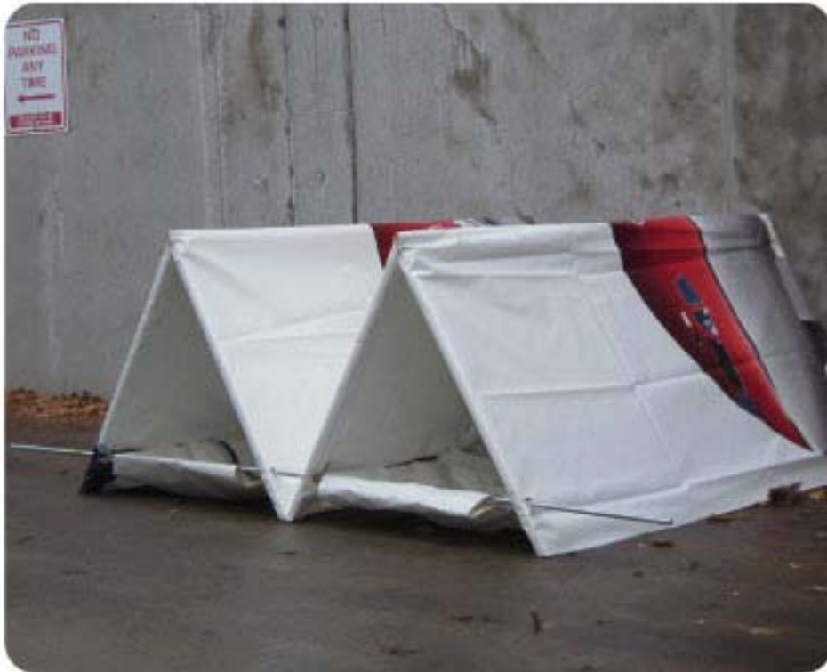
side view: note how hammocks are elevated by conduit and how water proof vinyl wraps around the entire form keeping the structure dry and reasonably weather tight.
